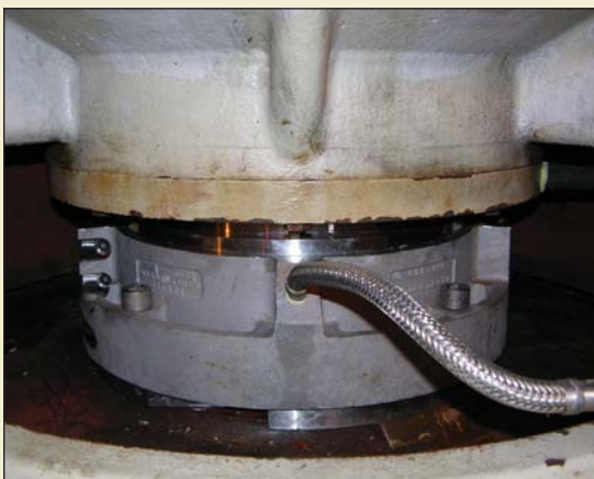
Split seal installation and repair are completed without equipment disassembly, saving time and operating costs.
